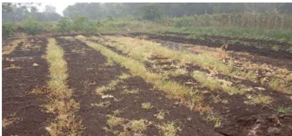
Figure 1. Land clearing activities
